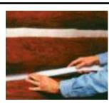
1. Install Grip Strip into caulk well of clean, stained logs.
