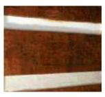
1. Start with logs that are stained with a coating compatible to Chinker's Edge (Sashco's Capture/Cascade or High Sierra Log Stain) and have properly installed backer material. (Avoid the use of blue or pink board.)
