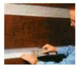
2. Tape the entire joint using mylar or duct tape.
