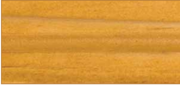
Wood was stained, then caulked.
