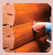
3 – Tool to ensure a tight seal to the top and bottom of the caulk line.
